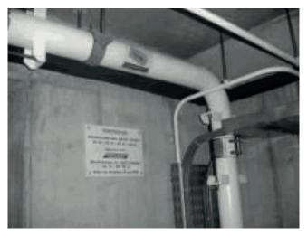
**Figure 3.** Abcite-coated piping after almost 20 years of use without any maintenance and in near-perfect condition. Image courtesy of Van Os-Duracoat, Belgium.
