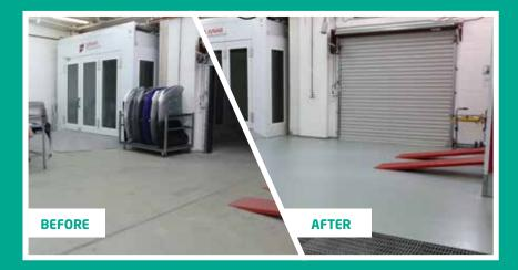
A highly durable and diverse coating, Corlar delivers outstanding corrosion and chemical resistance. It can be brushed, rolled or sprayed over a range of surfaces, including carbon steel, galvanised steel, stainless steel, aluminium, concrete, concrete block and wood, and it has an easy mixing ratio of 1:1 with Corlar hardener.
